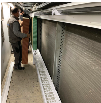
Easy and quick installation of the pads which are also easy to clean and replace.
