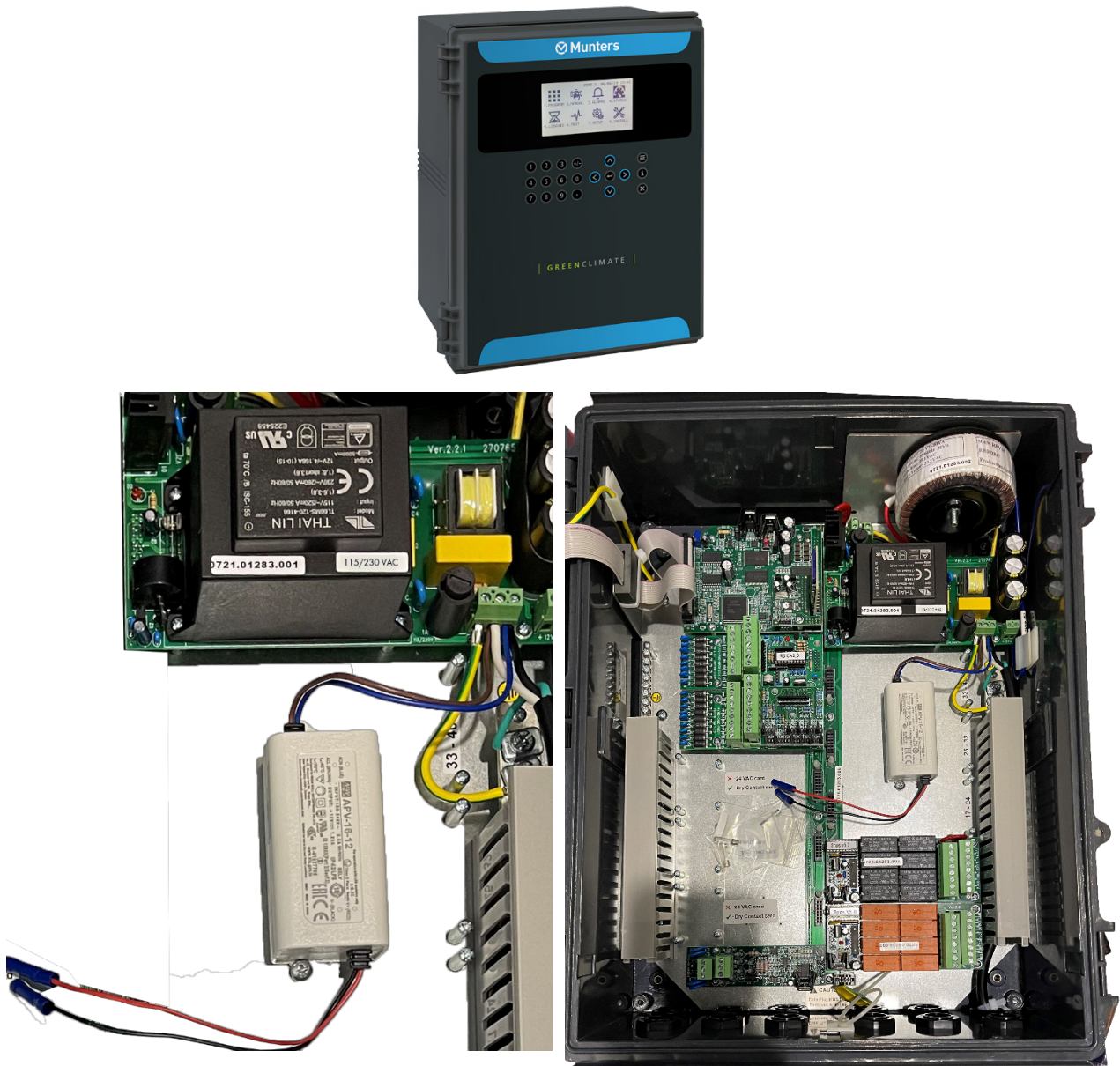
Figure 11: Wiring the CO2 Sensor Power Supply
