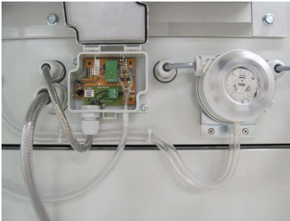
Figure 3.22 Connection for DPT (Reactivation fan)
