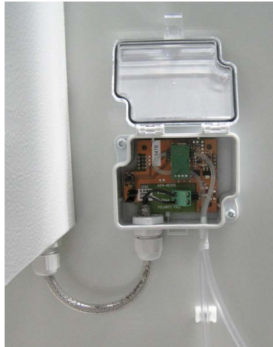
Figure 3.23 Connection for DPT (Process fan)
